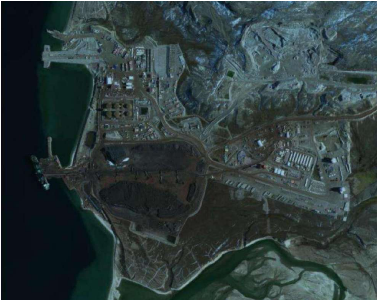
Mary River Mine - Aerial View of Milne Port - RCN, 2021
