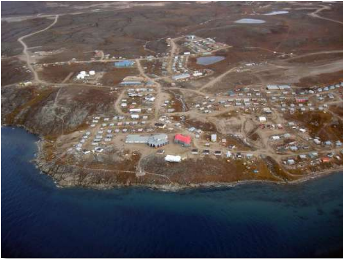
Pond Inlet - Aerial Shot - Camilla Desgagnés, 2007. Licensed under CC BY-SA 3.0
