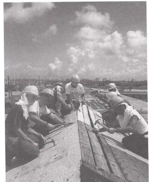
Canadian forces personnel repair some of the damage wrought by Hurricane Andrew in Florida.
